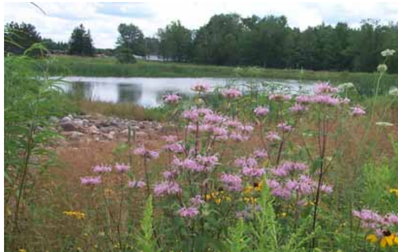
0.9 Acre Industrial Outlot Biofilter at Flambeau
