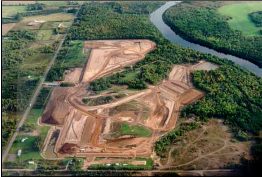
Flambeau Mine Site during construction.
