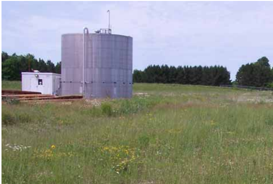
Reclaimed West Railroad Spur in foreground (Second year growth) in the Industrial Outlot at Flambeau
