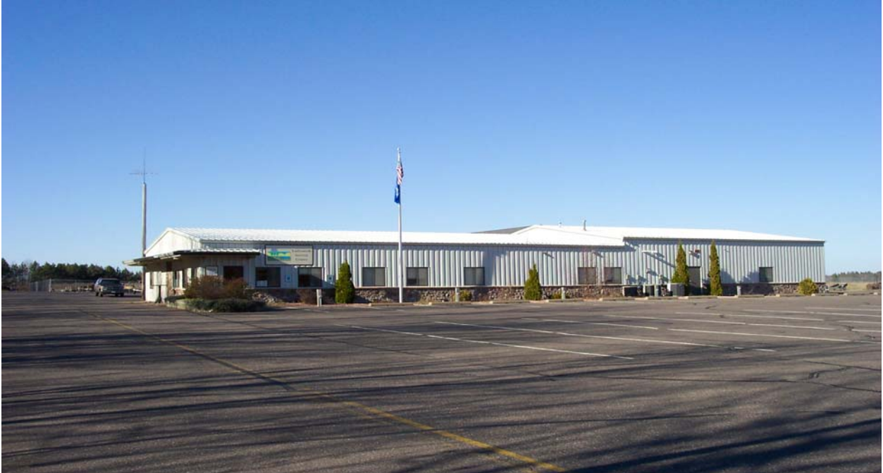
Figure 10.1 Wisconsin Department of Natural Resources Ladysmith Service Center
