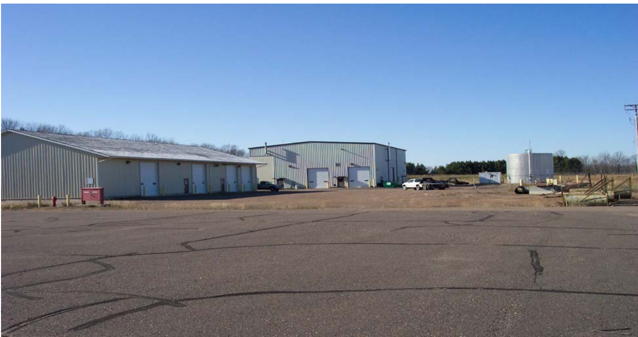
Figure 10.2 DNR Garage in Forefront and Xcel Energy Line Maintenance Garage
